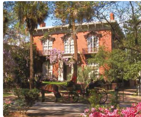
Mercer Home, Savannah Photo: Georgia Dept. of Economic Development
