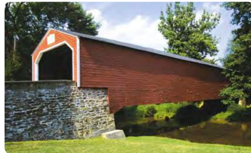
Covered Bridge Photo: Pennsylvania Tourism
